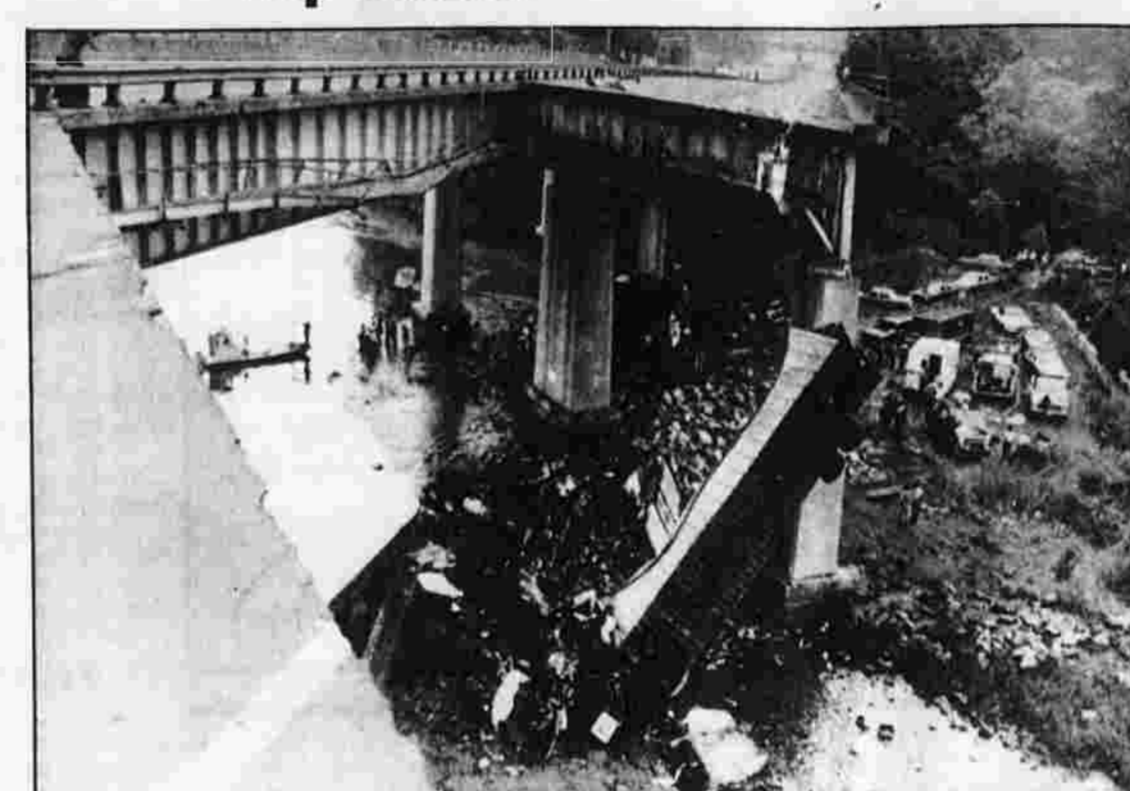
CONNECTICUT'S TOP STORY — The 1983 collapse of the Mianus River bridge was voted the top state story of the decade by editors and broadcasters.
